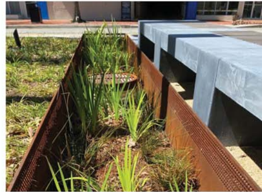
Rain gardens manage stormwater at the newly constructed pedestrian park.
